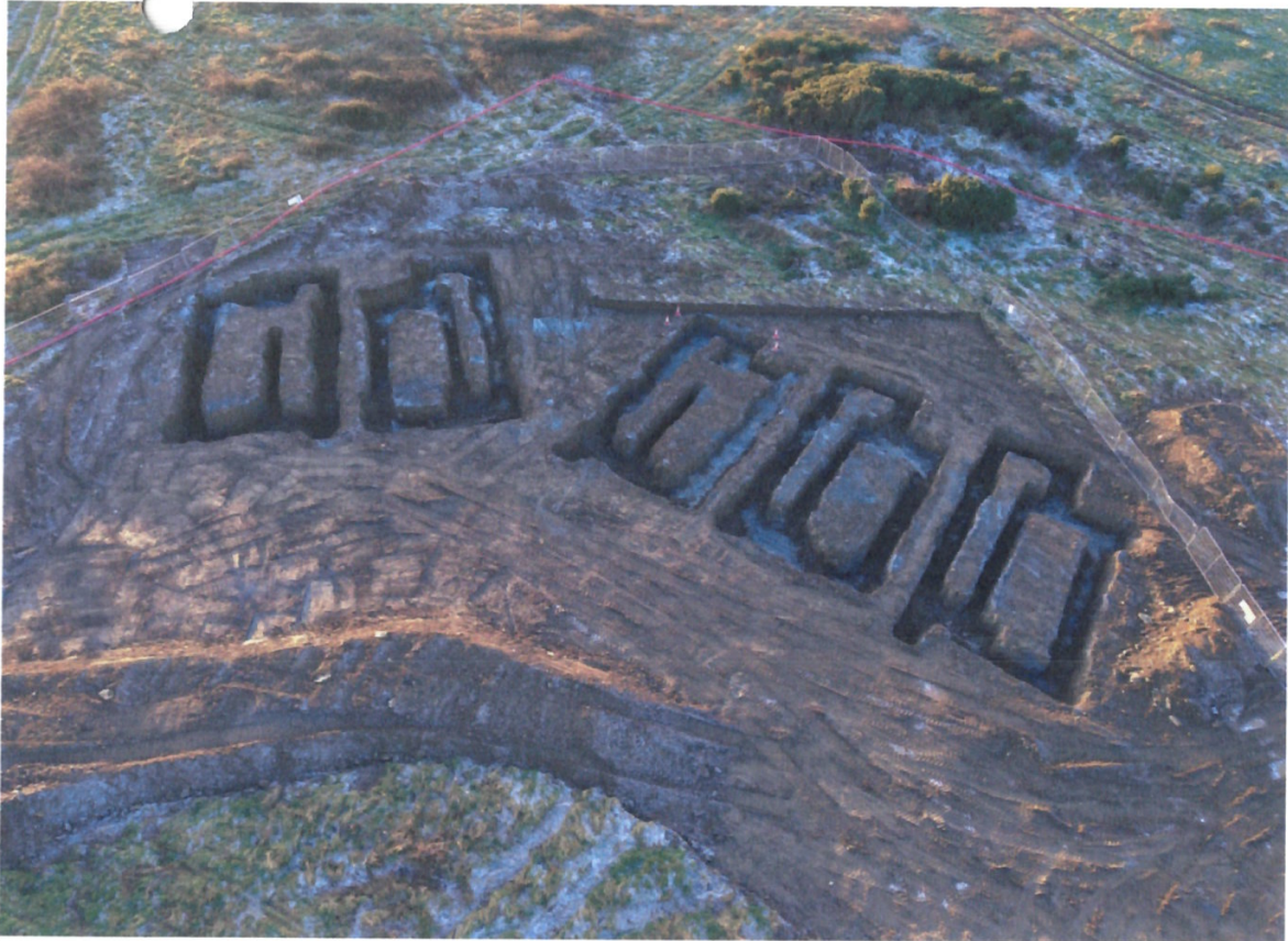
The foundation trenches for 5 units.
